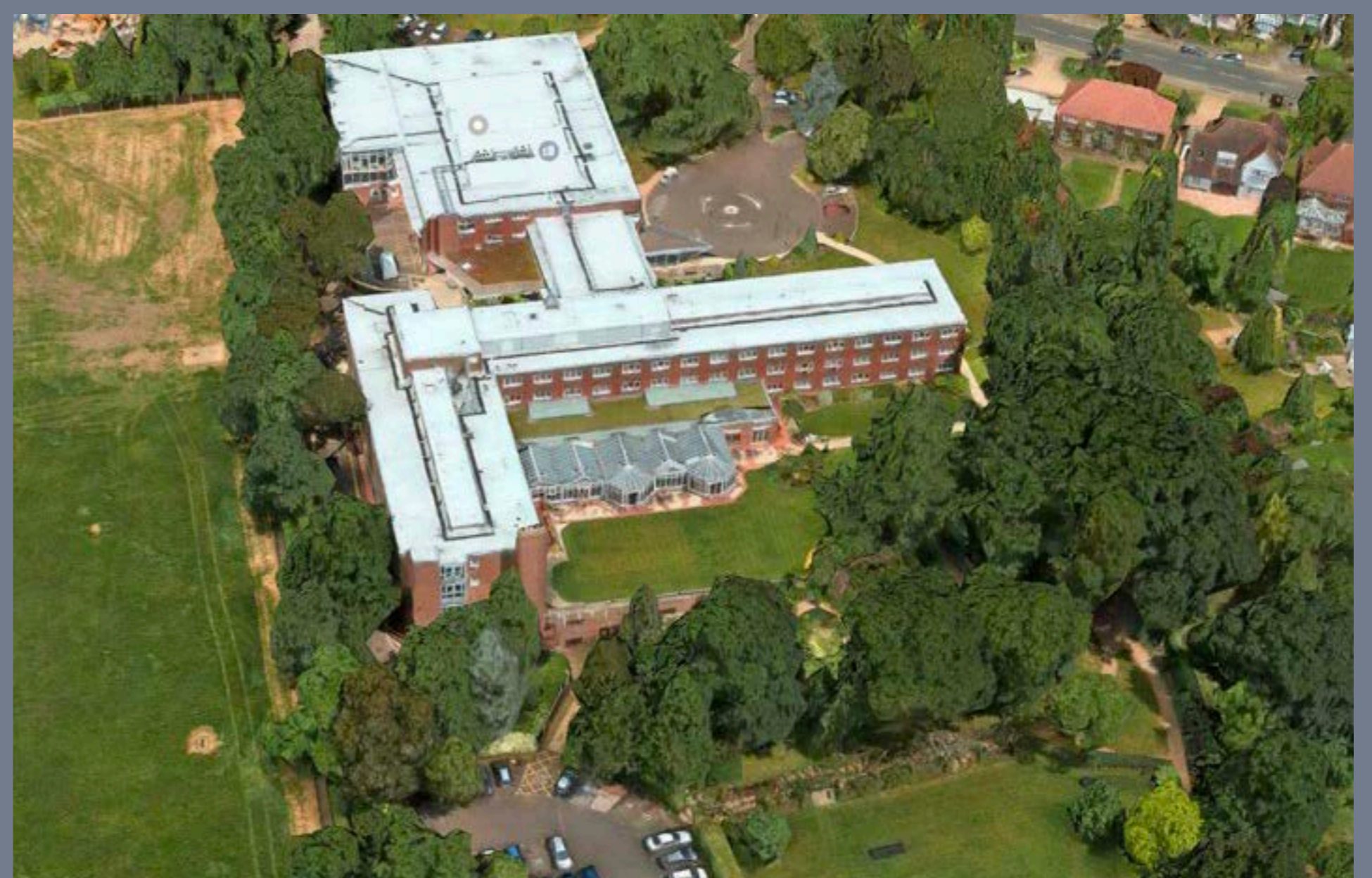
The existing Watch Tower House building
